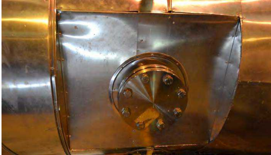
Illustration 13: Re-establishment of the Heat Insulation
